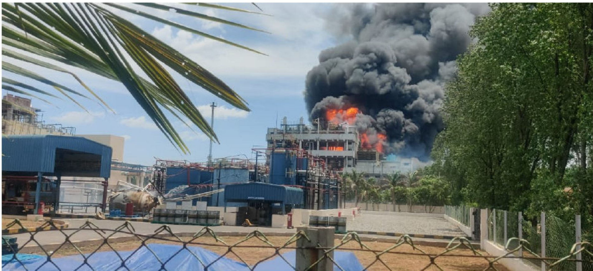
Fire broke out at SRS plant.
